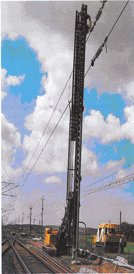
Figure 3a Lime cement installation instrument.
