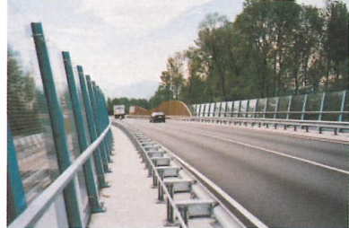
Acoustic barriers restrict noise propagation
