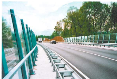
Acoustic barriers restrict noise propagation
