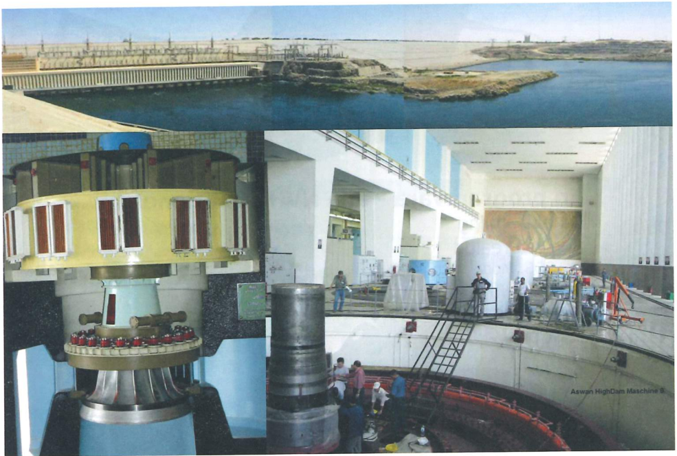
Fig.13: Aswan High Dam - site, model and power house with refurbishment of unit 9
