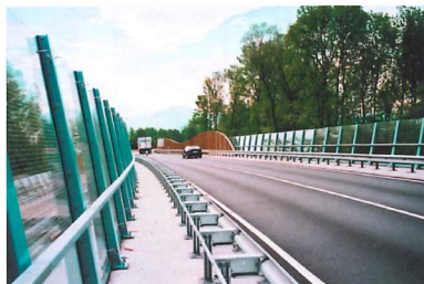
Acoustic barriers restrict noise propagation
