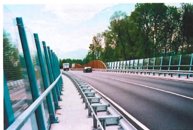
Acoustic barriers restrict noise propagation
