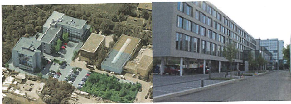
Figure 4. Müller-BBM in Planegg. a) The complex 1999, b) the latest building 2010.
